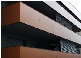
Phenolic panels and Fiber cement siding/cladding
